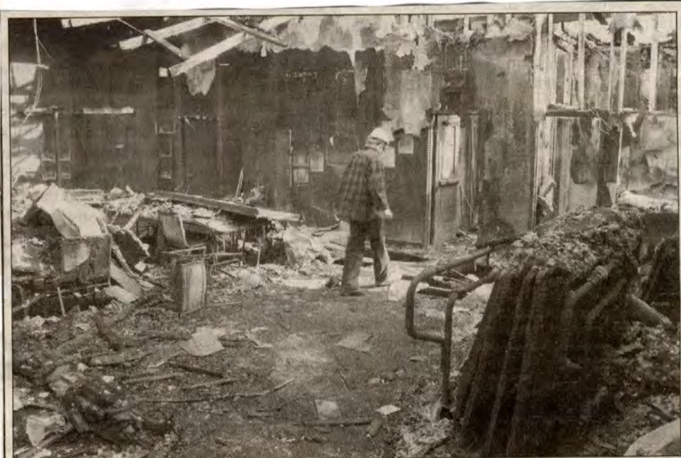
Taking out rubble
